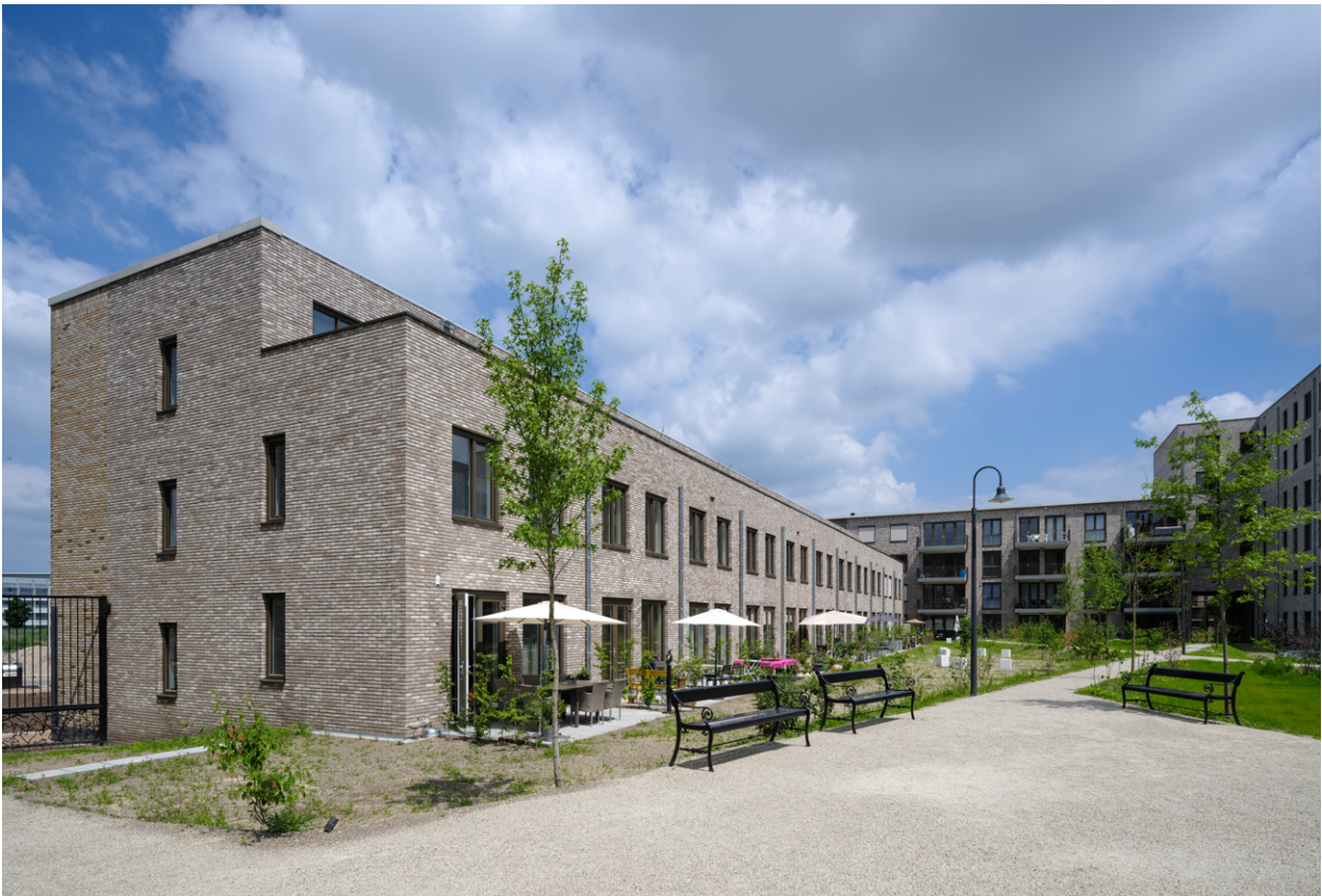
courtyard (left building A, middle building B)
