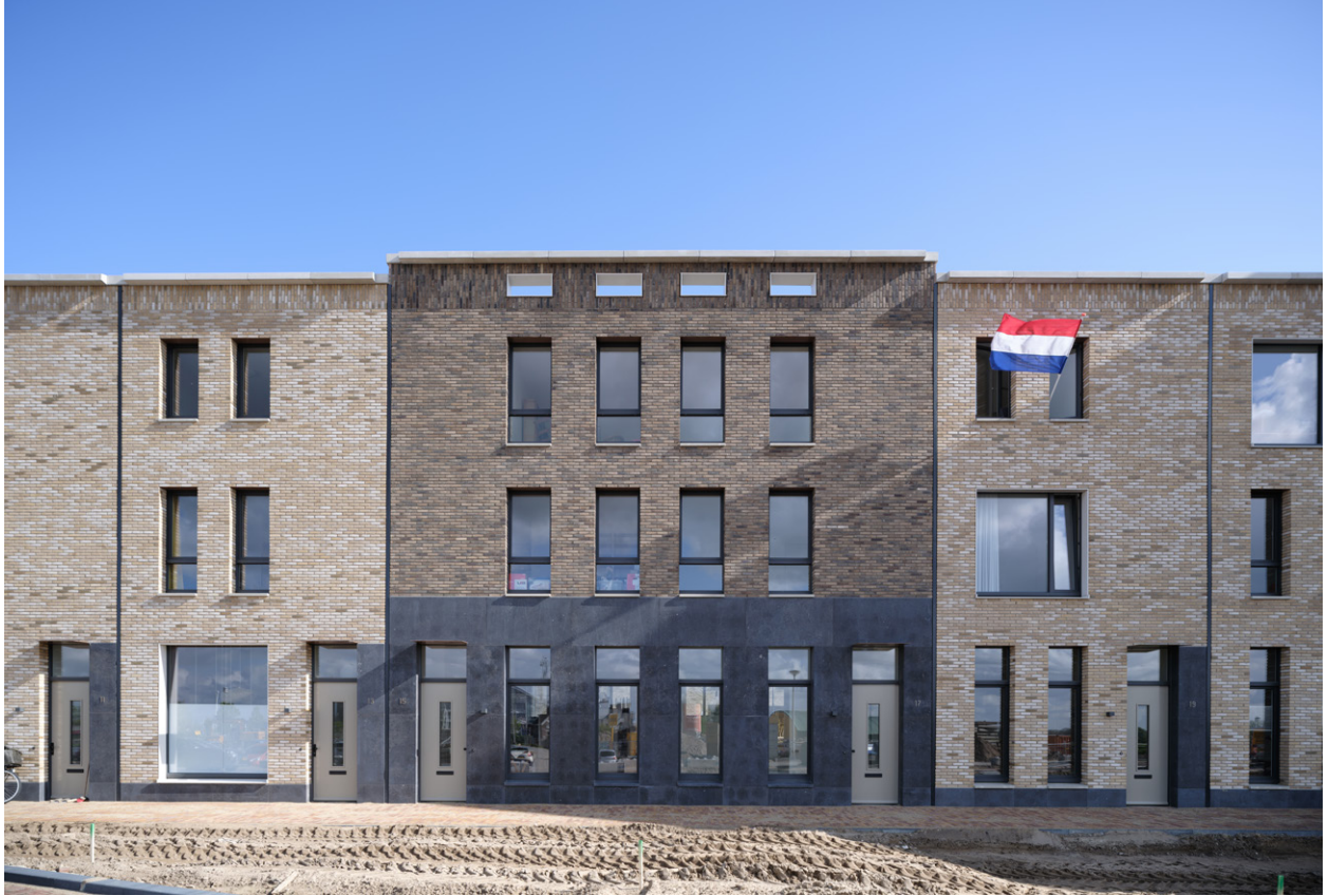
facade building A
