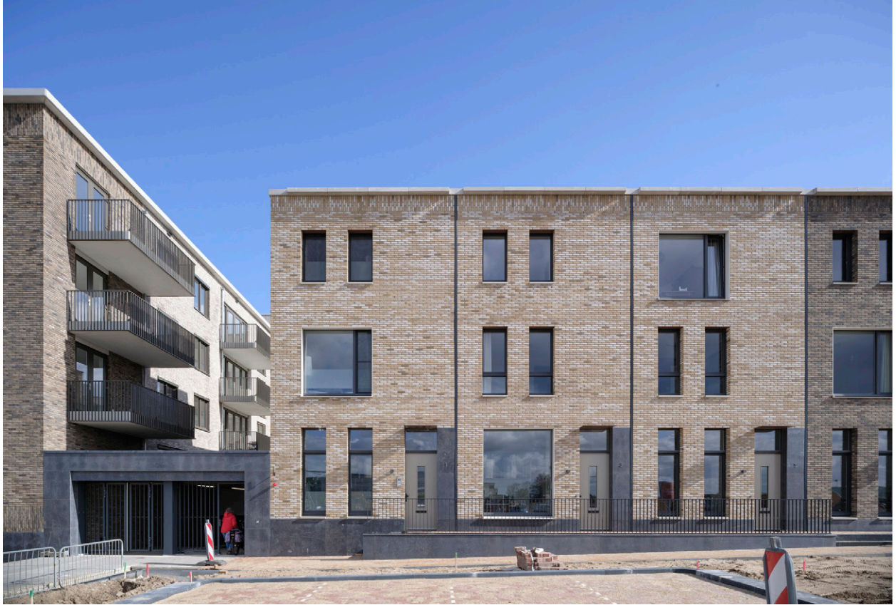
facade building A
