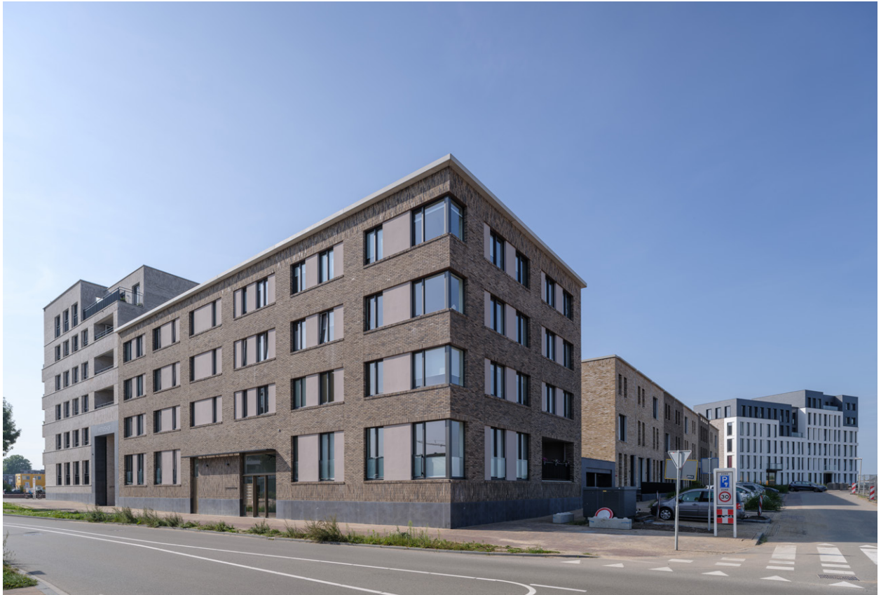
facade Coenensparkstraat building B
