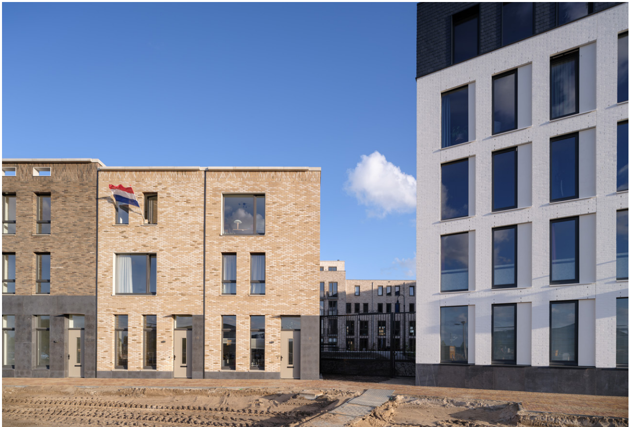
facade building A
