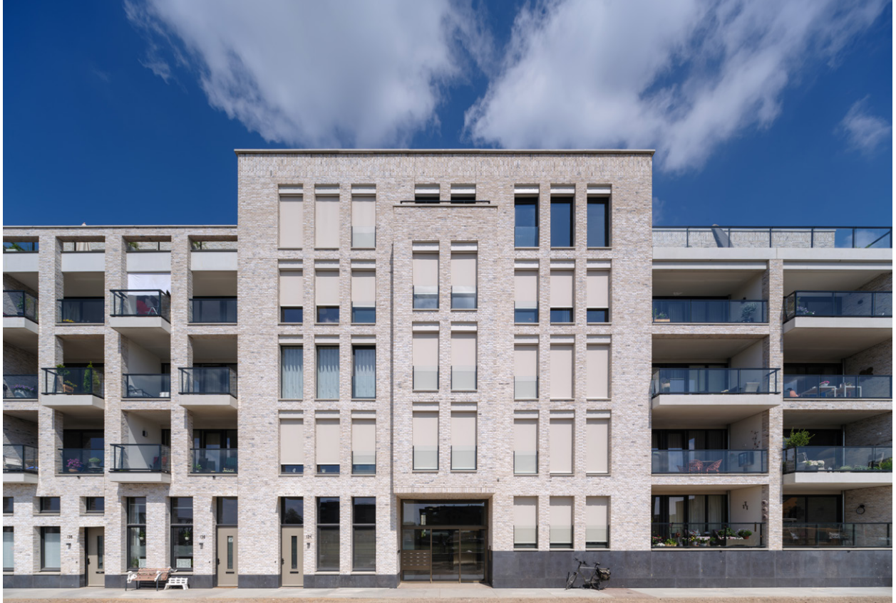
facade building E
