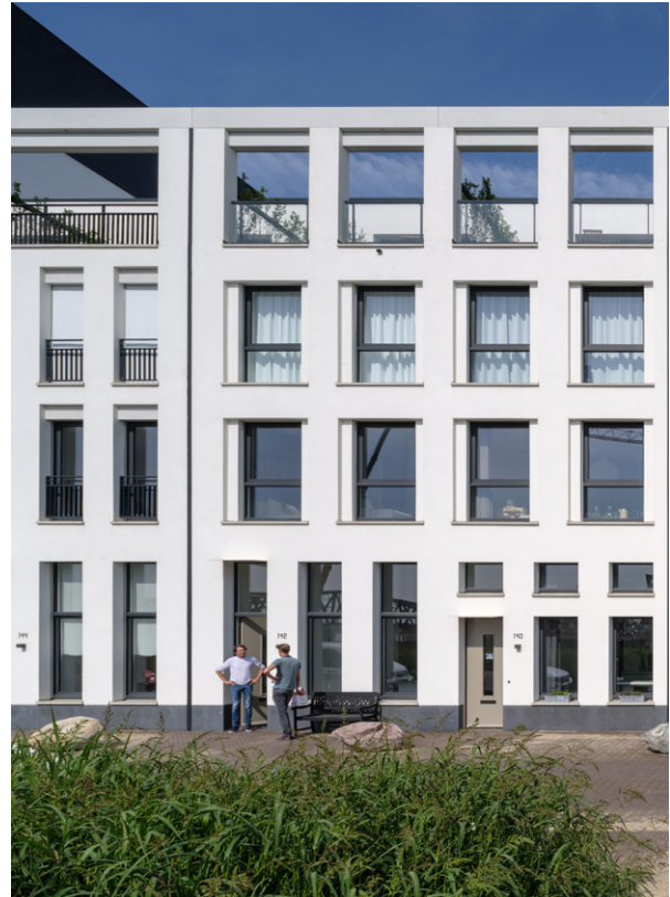
facade building F
