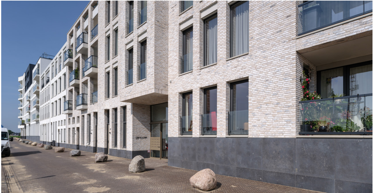
facade building E
